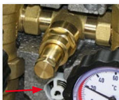
(3) Check valve position when it is supplied.
